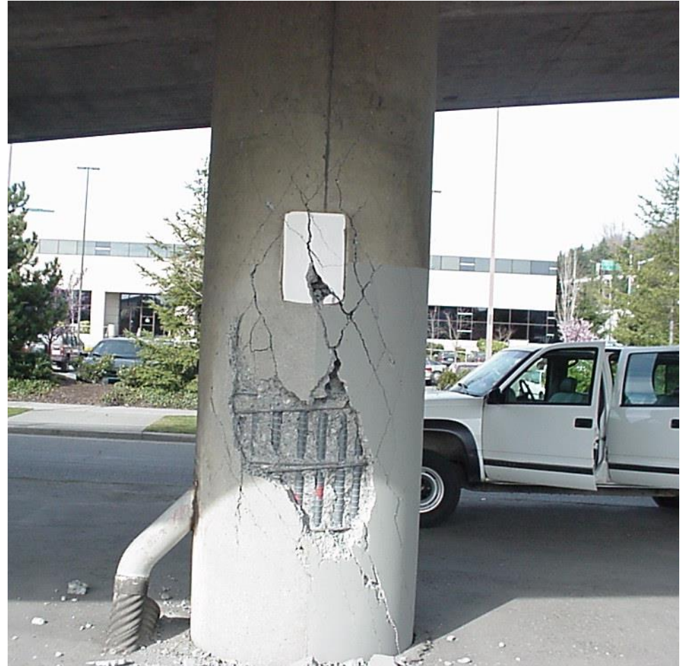
I-5 Beacon-Holgate Bridge in Seattle
